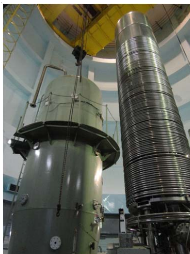
High Voltage Column of FOTIA
